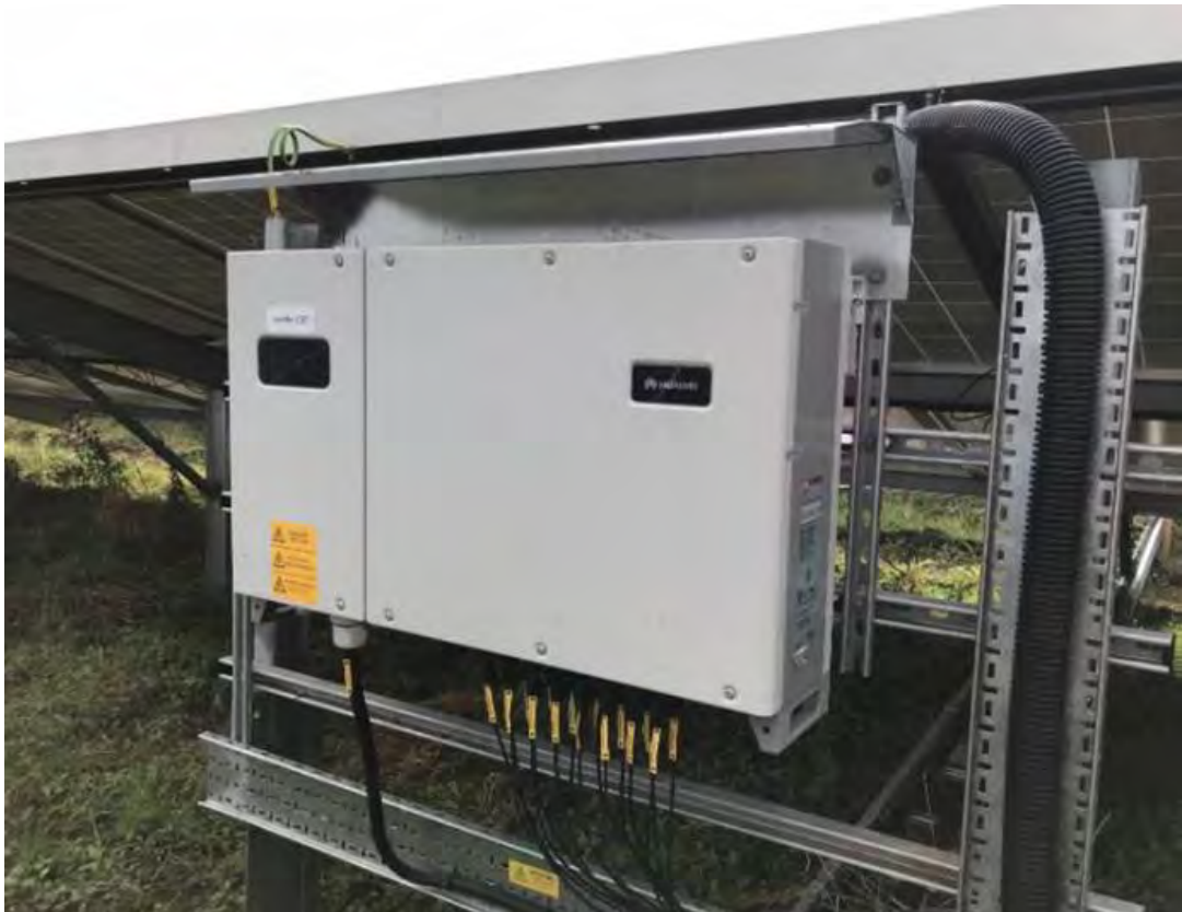
Figure 5 Typical String Inverter (image reproduced courtesy of Huawei)
