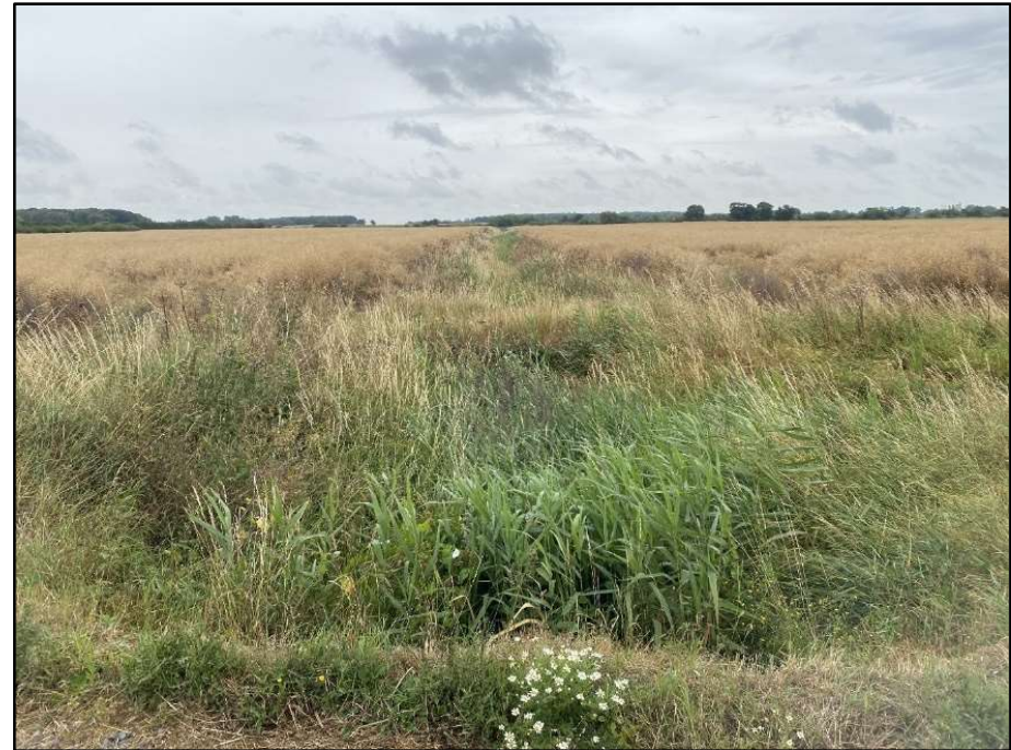
Location: 42 NGR: TF 14977 49425 Photo Date: 14 July 2023 Description: Unnamed drain, with overgrown vegetation throughout channel, left bank c.1m, right bank c.1m, width c.3m. Facing east.
