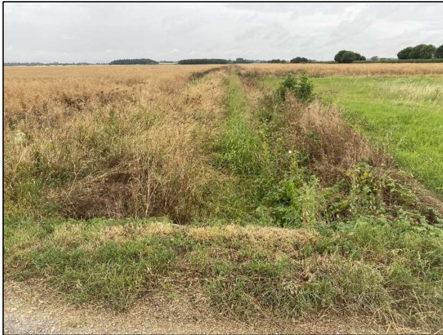
Location: 41 NGR: TF 15070 49249 Photo Date: 14 July 2023 Description: Unnamed drain, with overgrown vegetation throughout channel, left bank c.1m, right bank c.1m, width c.3m. Facing west.
