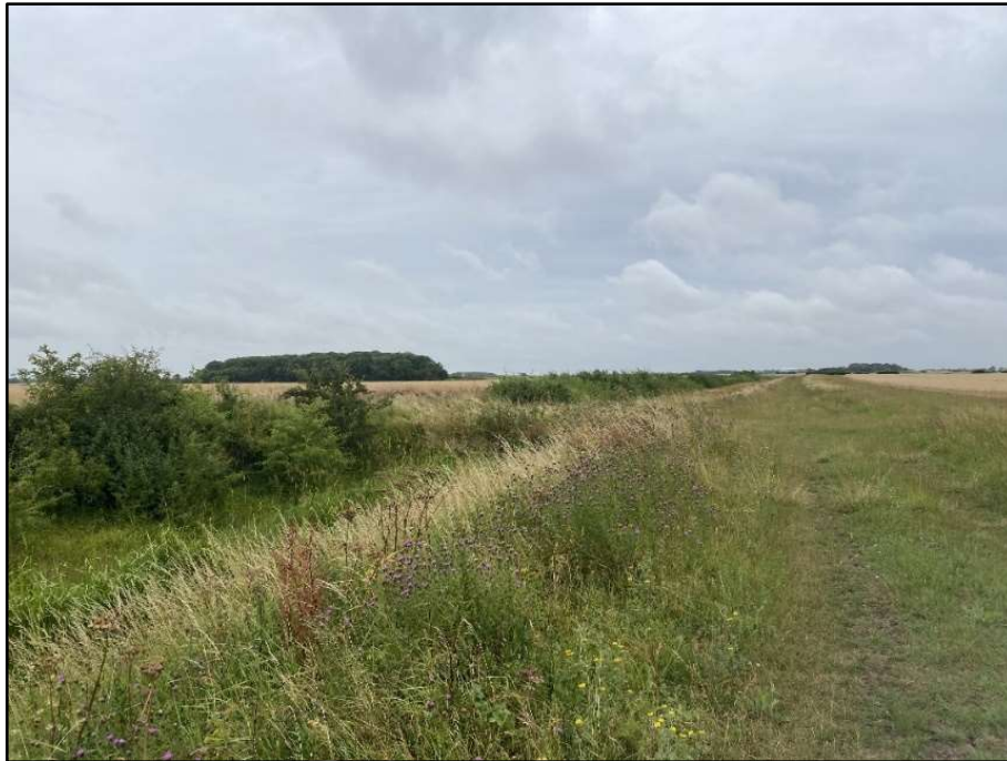
Location: 31 NGR: TF 14539 48488 Photo Date: 14 July 2023 Description: Passing place and unnamed drain, with hedge and overgrown vegetation throughout channel, left bank c.1.5m, right bank c.1.5m, width c.4m. Facing southeast.
