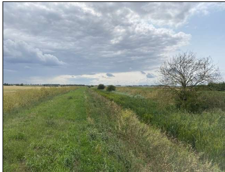
Location: 14 NGR: TF 15817 48268 Photo Date: 13 July 2023 Description: Unnamed drain, with overgrown vegetation throughout channel, left bank c.1.5m, right bank c.1.5m, width c.2m. Facing west.
