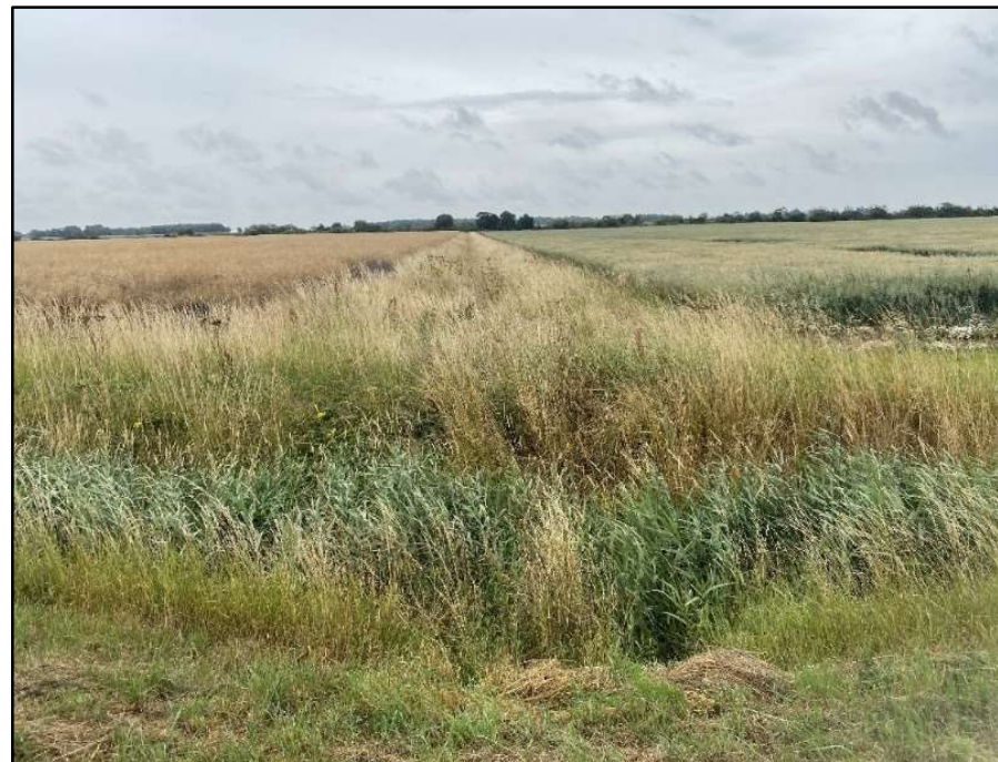
Location: 40 NGR: TF 15041 49314 Photo Date: 14 July 2023 Description: Unnamed drain, with overgrown vegetation throughout channel, left bank c.1.5m, right bank c.1.5m, width c.2m. Facing east.
