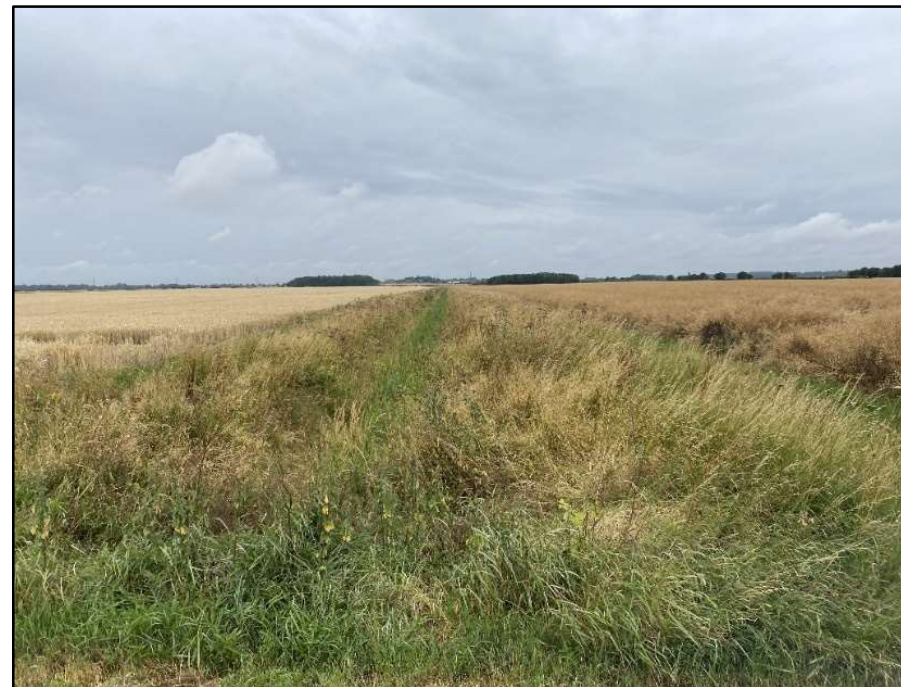
Location: 38 NGR: TF 15149 49098 Photo Date: 14 July 2023 Description: Unnamed drain, with overgrown vegetation throughout channel, left bank c.1.5m, right bank c.1.5m, width c.4m. Facing west.
