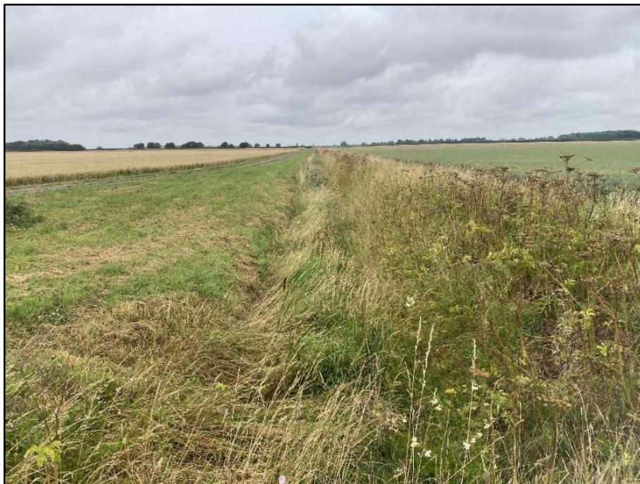
Location: 37 NGR: TF 15218 48969 Photo Date: 14 July 2023 Description: Passing place and unnamed drain, with hedge and overgrown vegetation throughout channel, left bank c.1.5m, right bank c.1.5m, width c.2m. Facing north.
