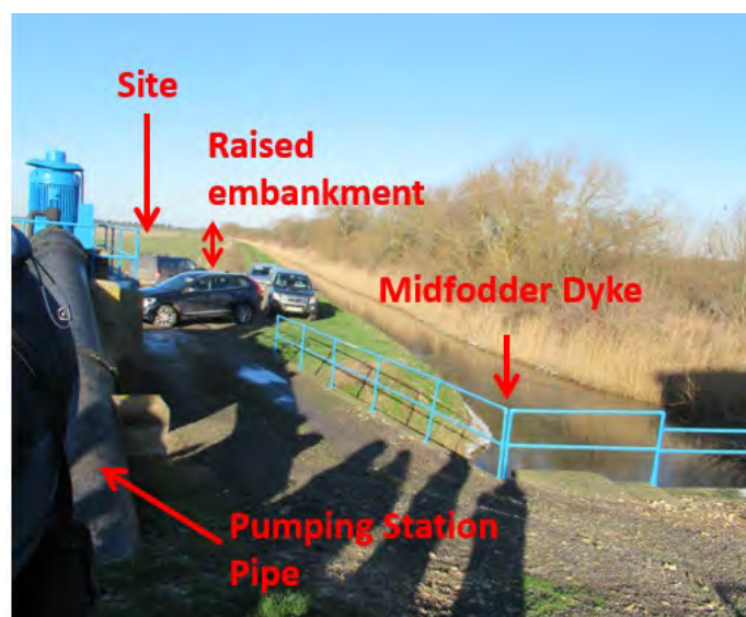
Figure 7. Midfodder Dyke (looking north from Ewerby Pumping Station)
