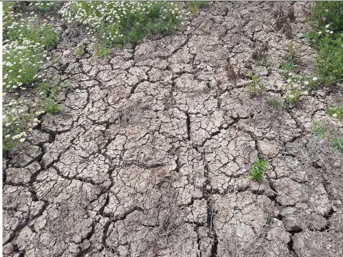
Figure 2. Desiccation cracks within footpaths.
