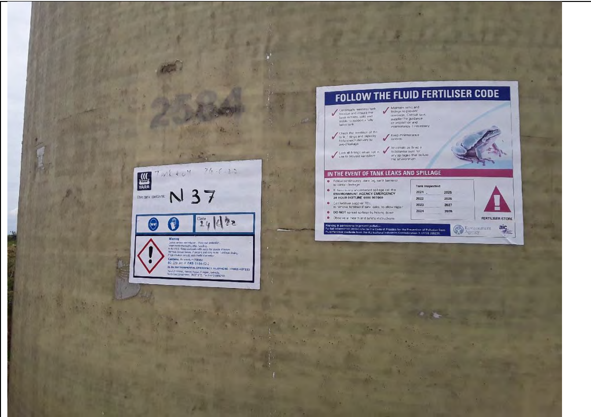
Figure 13. Chemical labels on the above ground storage tank in the centre of the Solar Array Area.
