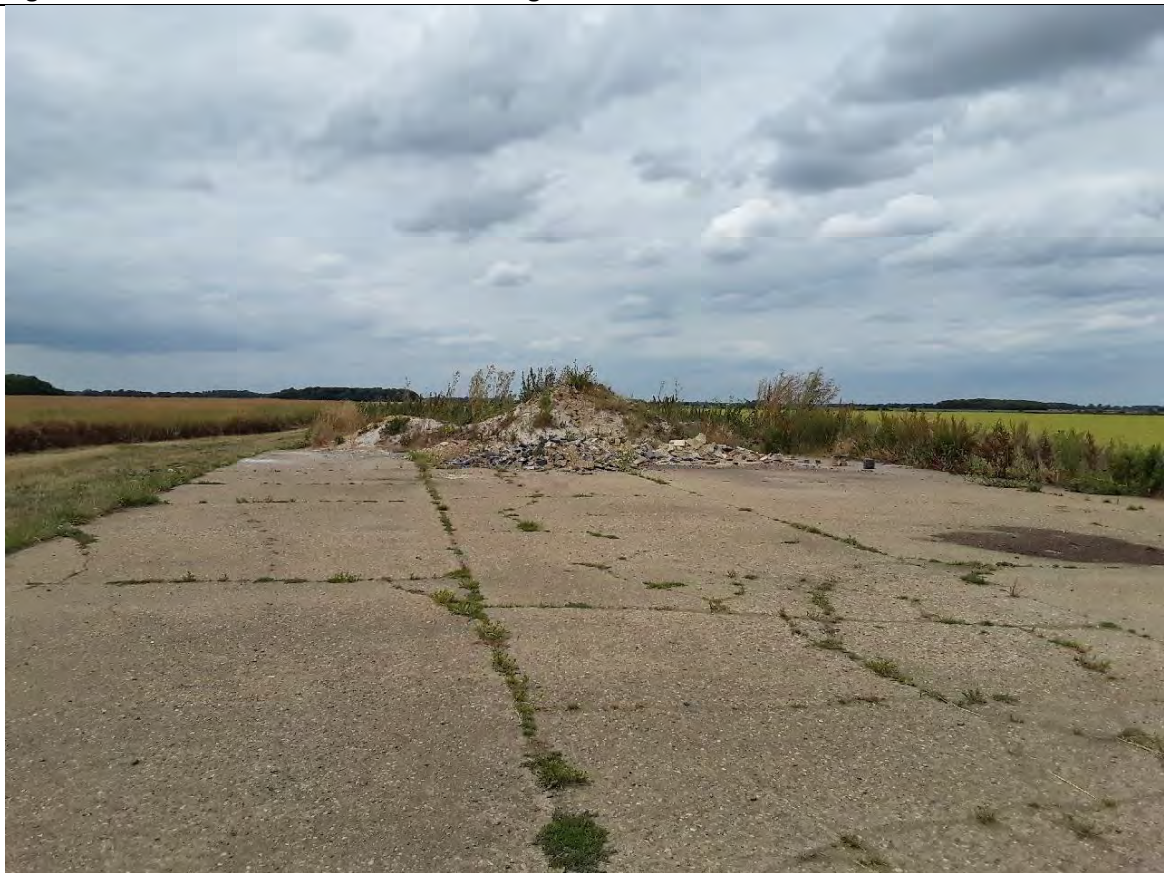
Figure 18. Area of hardstanding in the south of the Solar Array Area.
