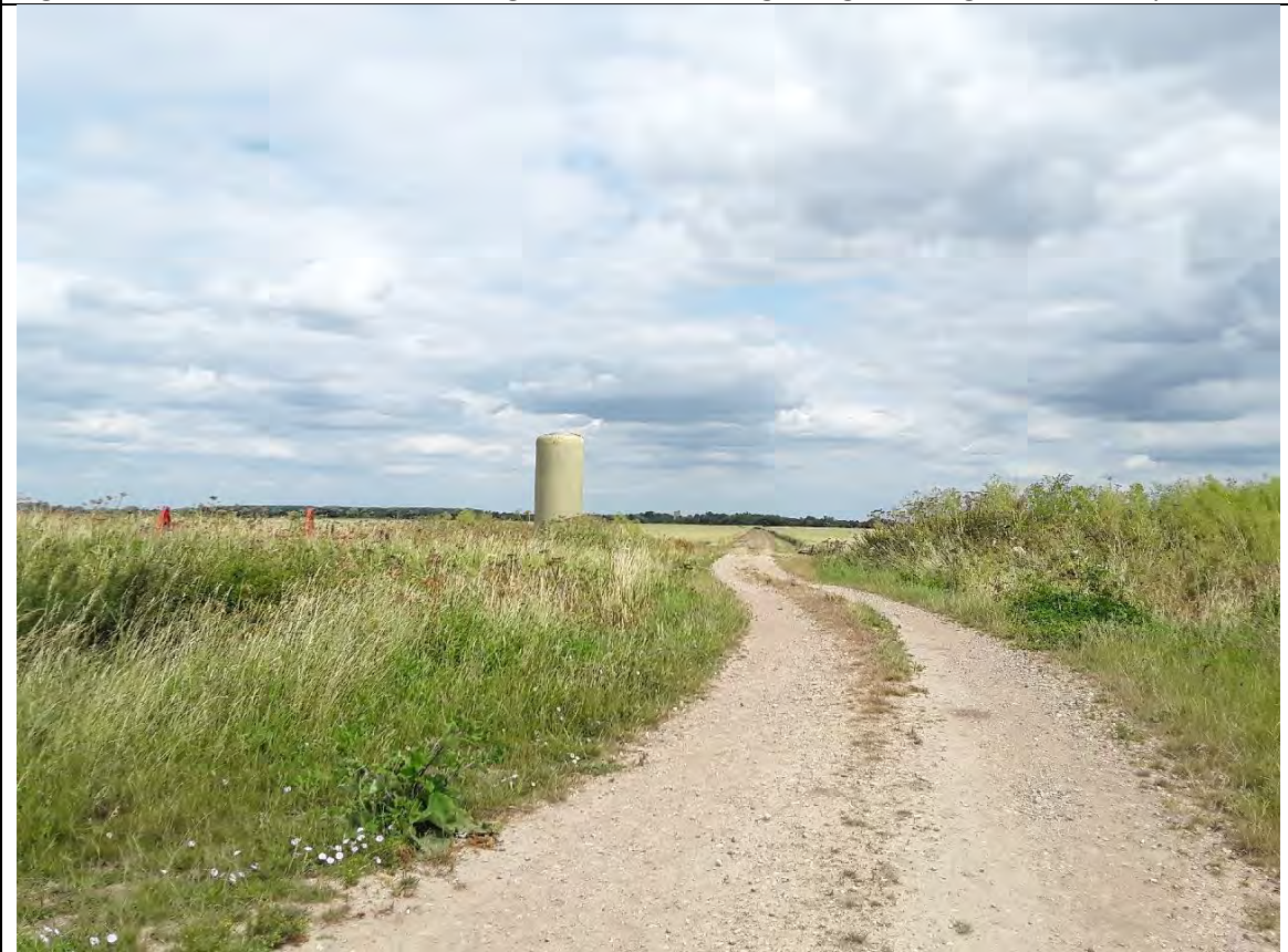
Figure 12. View looking east along the access track in the centre of the Solar Array Area, showing the storage tank.
