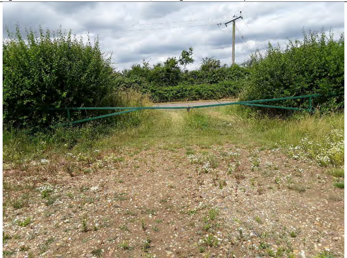
Figure 10. Showing a gated access point into the north of the Site suitable for vehicles.
