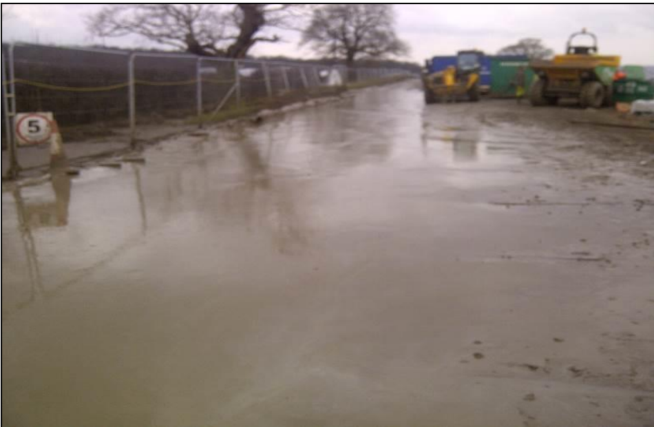
Condition Mid construction
